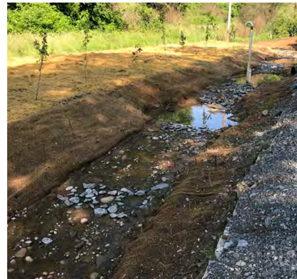
Impacted Stream Post Construction
