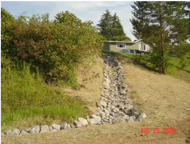
Erosion Repair – Rip Rap Armored Ditch
