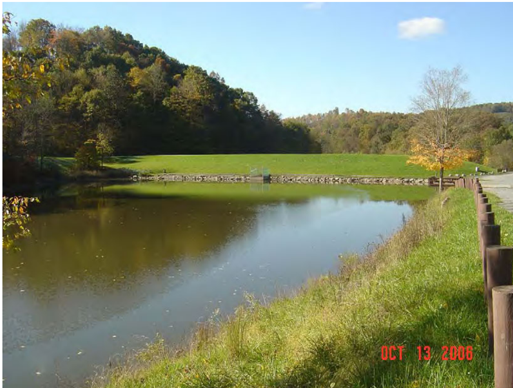
JIMMY LEWIS DAM MODIFICATION, MERCER CO., WV
