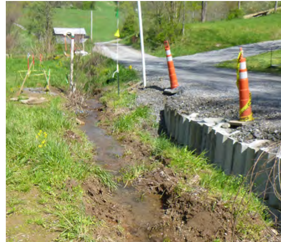
Impacted Stream Before Construction
