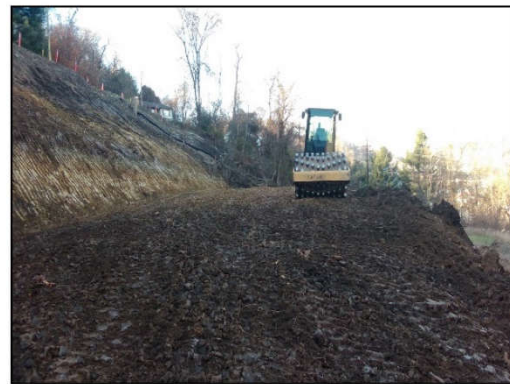
During Construction of Repair
