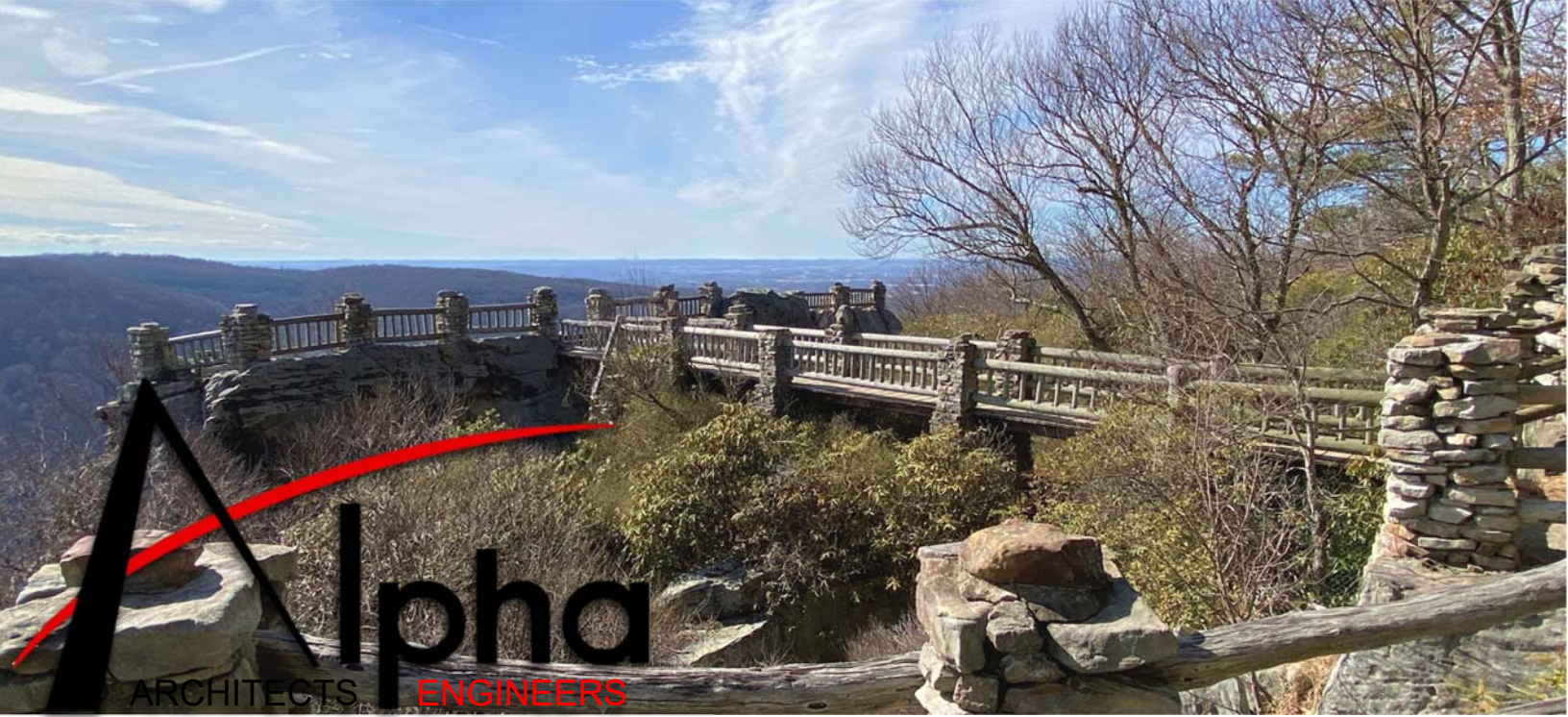
Coopers Rock Pedestrian Bridge Evaluation - 2022
