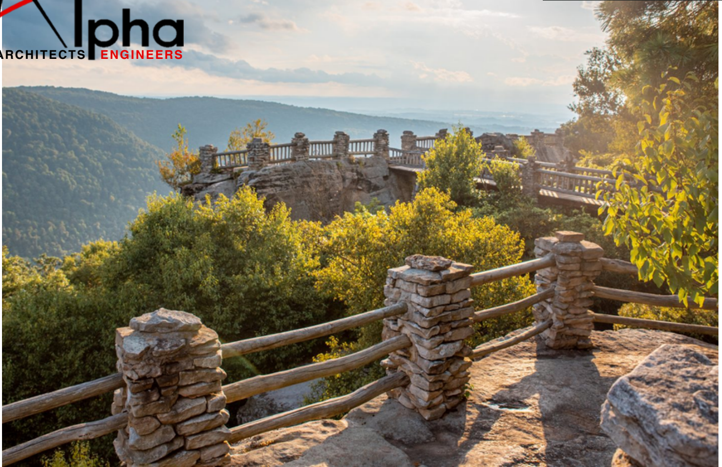
Cooper's Rock State Park Pedestrian Bridge
