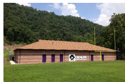
Riverview Field House - Locker Rooms & Bathrooms
