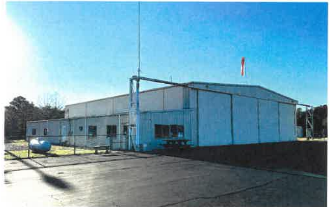
Existing Terminal/Hangar Building
