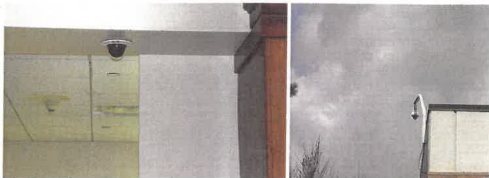
About 200 Bosch cameras are installed throughout Highland-Clarksburg Hospital. NIN-733 Flex-idome Starlight HD 720p models were used for the interior. VG5-7000 series pan/tilt/zoom (p/t/z) cameras provide coverage of external areas and parking lots.
