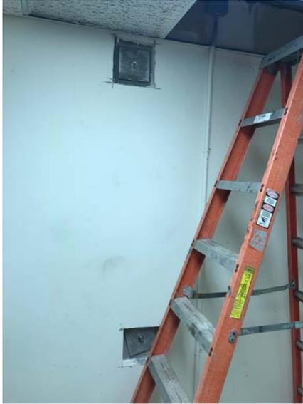
3<sup>rd</sup> floor with exterior steel frame thru-bolts visible.
