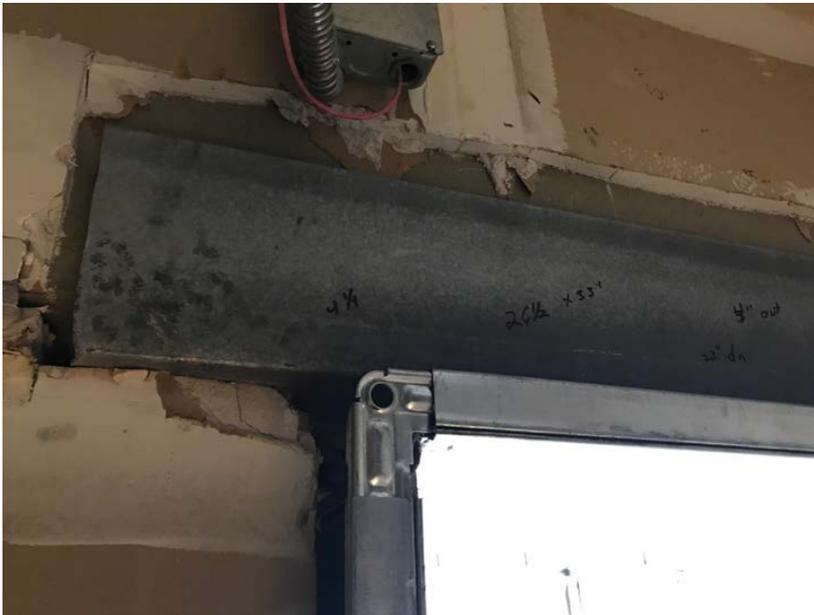
Interior view of the lintel above duct penetration at 3<sup>rd</sup> floor.
