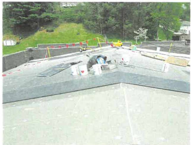
Roof repair on the Coal Heritage Discovery Center in Mt. Hope.
