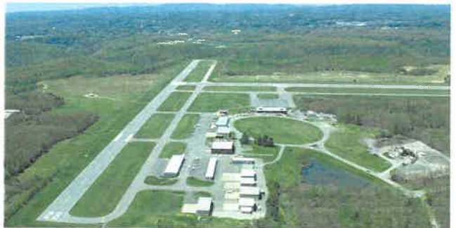
Raleigh County Airport runway rehabilitation.
