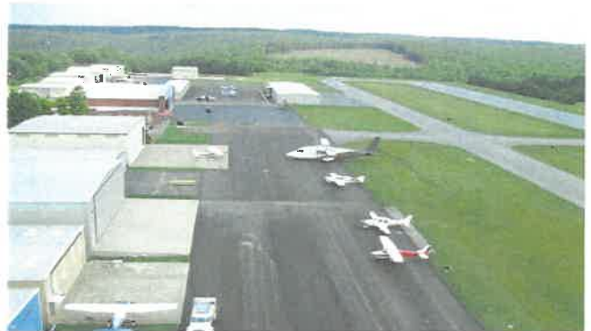
Raleigh County Airport apron repairs and improvements.
