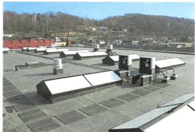
Roof repair on the State Road Commission Building in Charleston.
