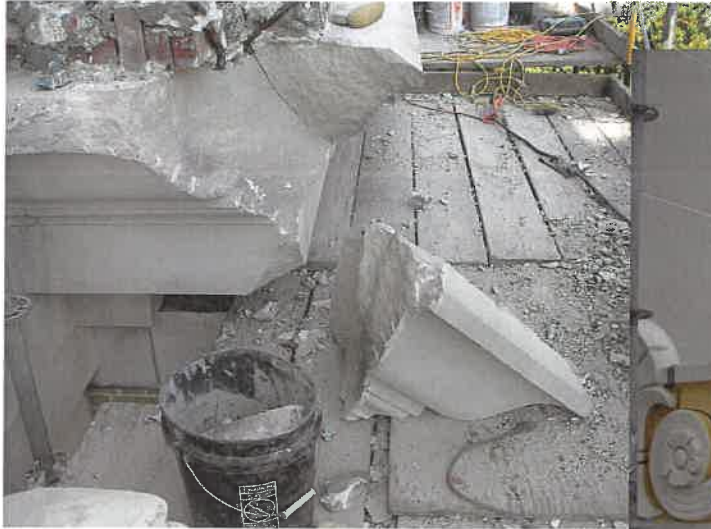
Portions of the limestone cornice were damaged to the point that they fell when work was being conducted and had to be pinned back in place.
