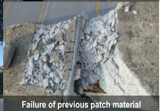
Full-depth Slab Repair
