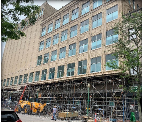
West Virginia Diamond Building – temporary protection for pedestrians while maintaining building occupancy.
