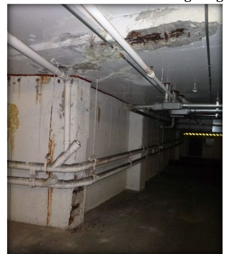
Corrosion damage on reinforced concrete column at basement wall
