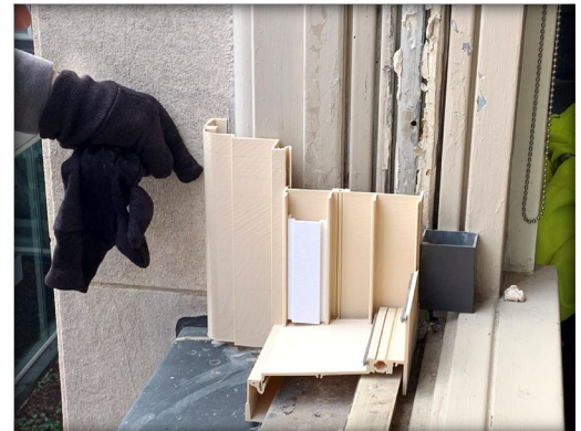
3D-printed window prototype used to verify complex historic window replica profiles
