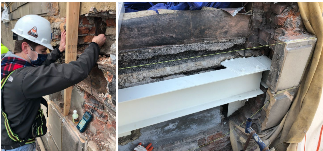
Ultrasonic Pulse Velocity Measurement of Corroded Structural Steel to Evaluate Reduced Capacity [left] and Structural Member Replacement [right]
