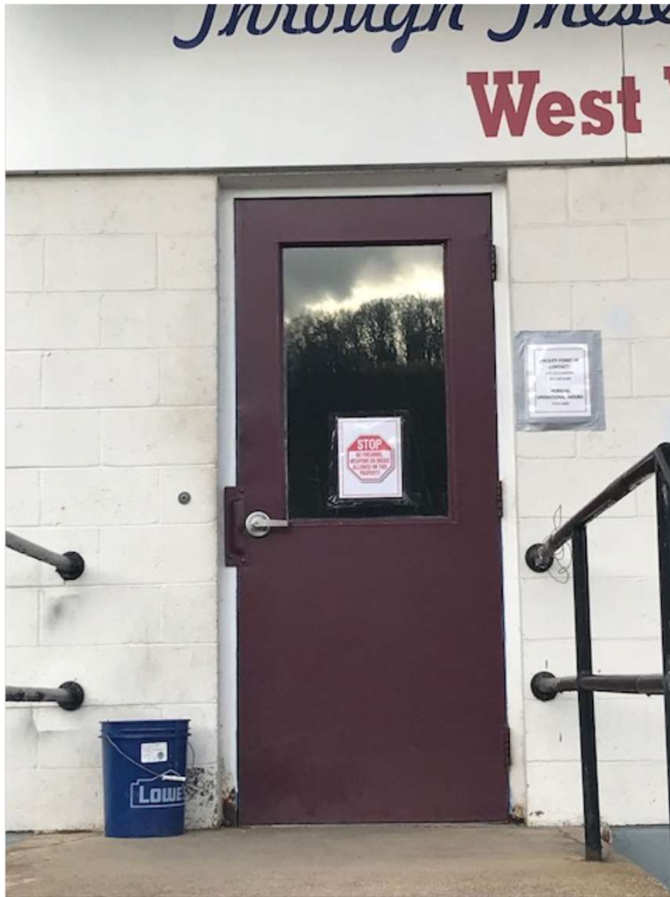
Main Entrance New Install Photo 1
