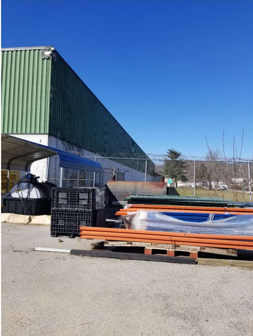
CCTV Outdoor Camera Locations (Front Side of Building Right of Entrance)
