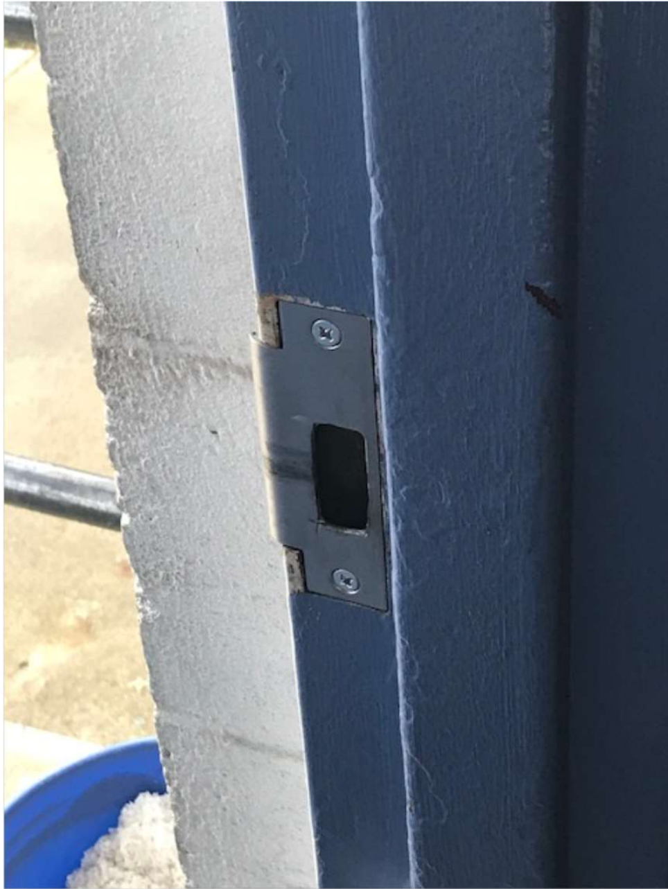
Main Entrance New Install Photo 2
