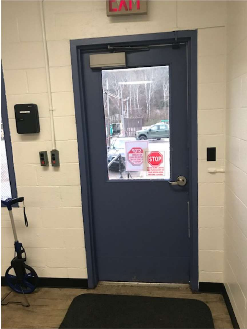
Main Entrance New Install Photo 3
