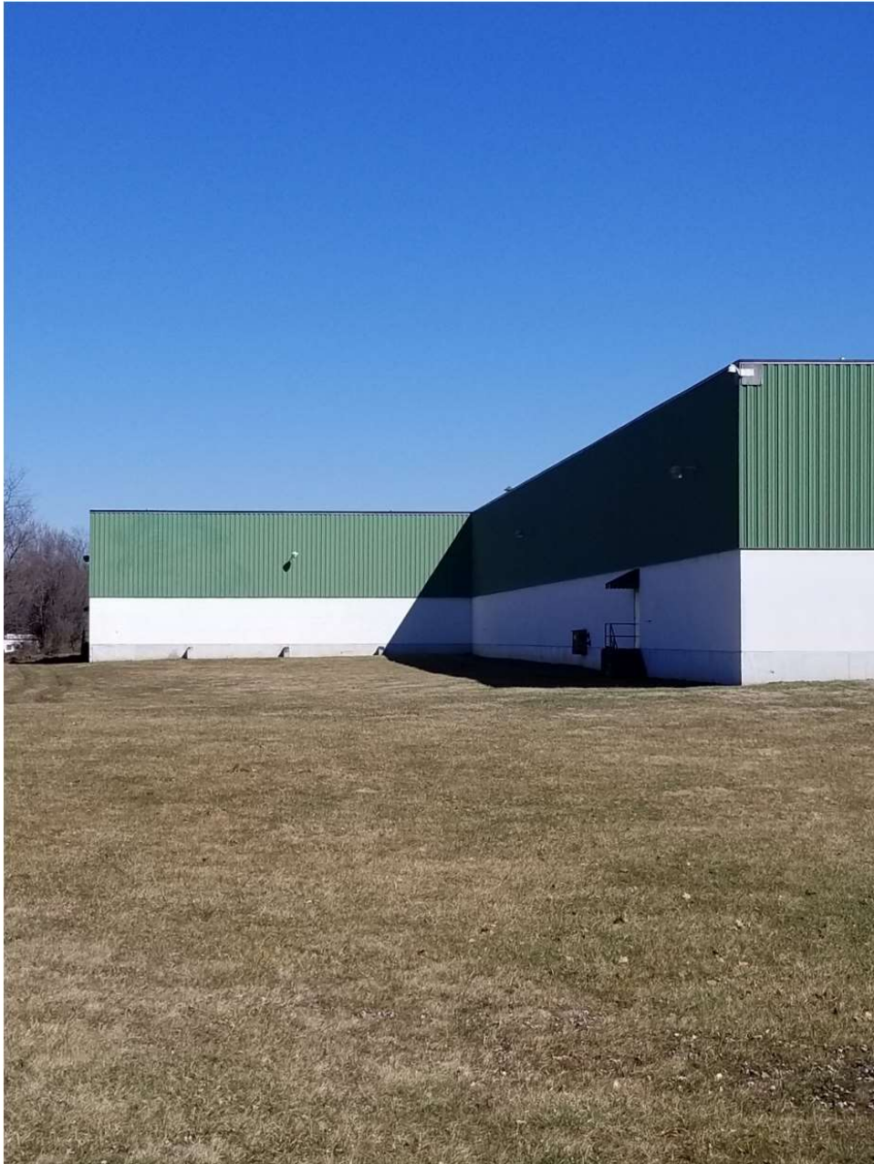
View of Left Side to Rear View of Building
