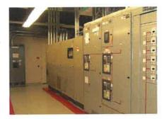
cabling cabinets to adapt input and output connections from existing infrastructure to new equipment.
