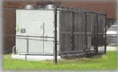
Chiller & Air Handling Unit Renovations
