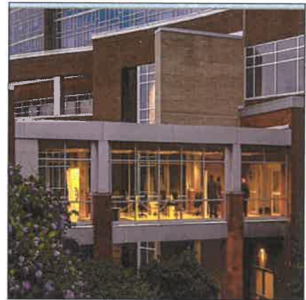
United Hospital Center Breezeway
