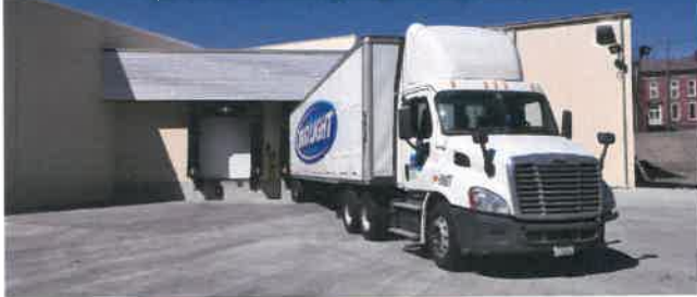
After Views of Carenbauer Building Addition (at the site of Sterling Drug Building Demo)
