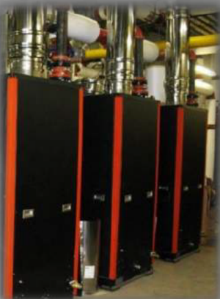
Condensing Hot Water Boilers
