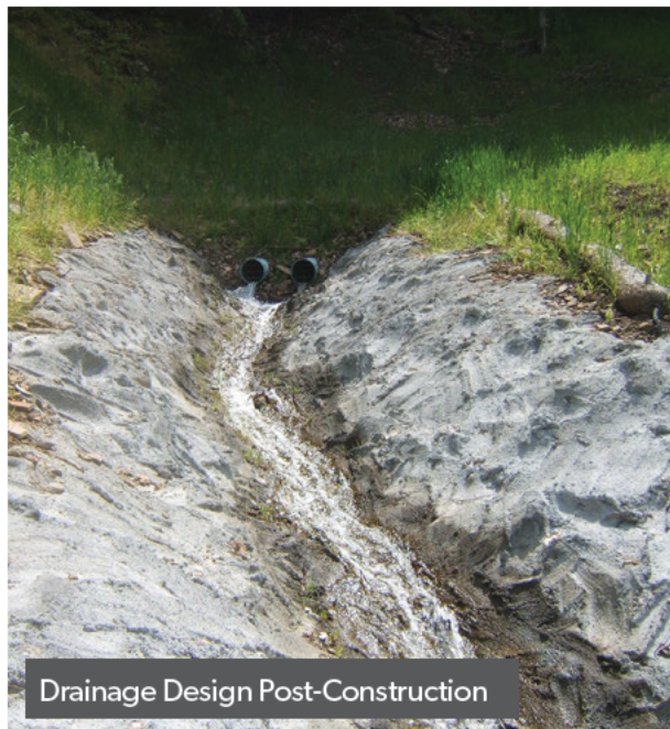
Drainage Discharging into a Stormwater System
