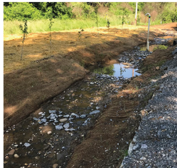
Impacted Stream Post Construction
