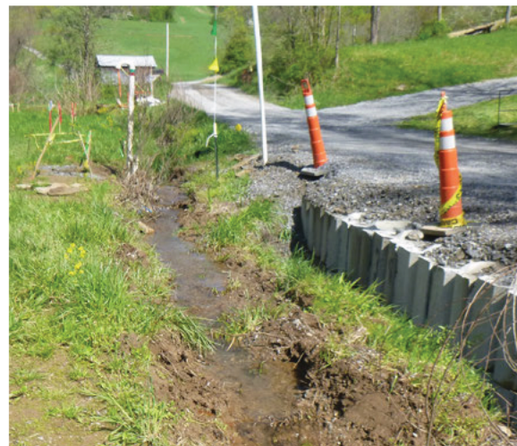
Impacted Stream Before Construction
