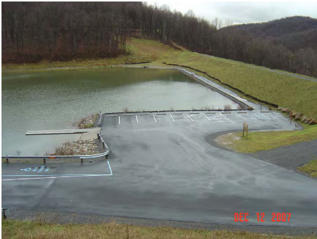
BAILEY DAM MODIFICATION, MONONGALIA CO., WV
