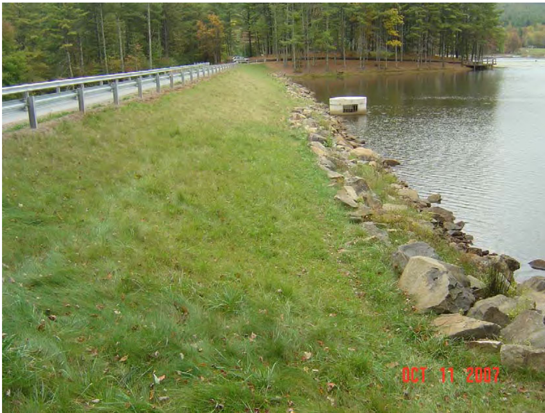
MONCOVE DAM MODIFICATION, MONROE CO., WV
