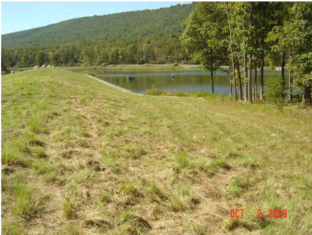
WARDEN LAKE DAM MODIFICATION, HARDY CO., WV
