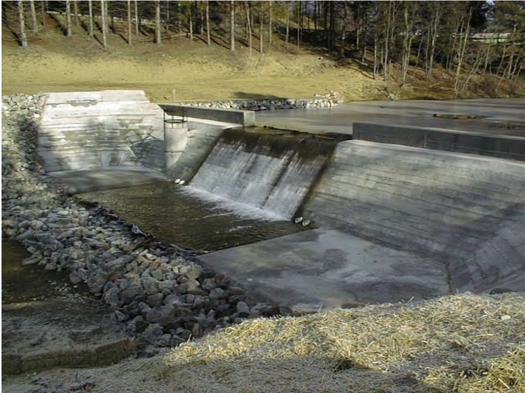
THOMAS DAM MODIFICATION, THOMAS, WV
