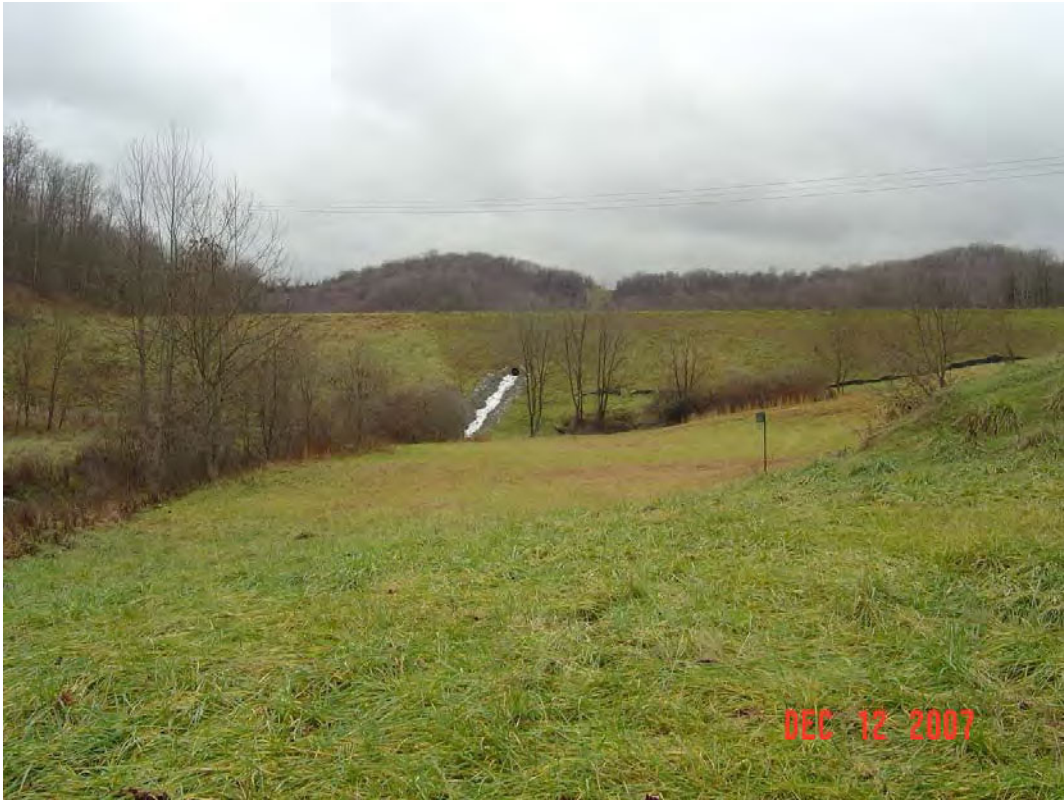
LEMLEY DAM MODIFICATION, MONONGALIA CO., WV
