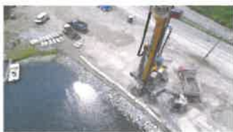
Drilling a soil-cement column at East Reservoir.
