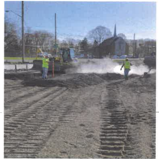
RCC Placement at North Reservoir Dam East Embankment
