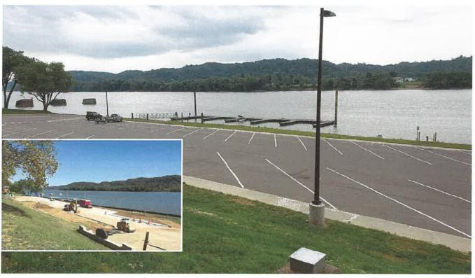
E.L. Robinson Engineering is responsible for project planning, permitting, design, and construction management of Riverfront Access Improvements for the City of Gallipolis, Ohio. The project provides upgrades to the existing river access including a new access road, 37 additional boat trailer parking spaces with make ready and tie down areas, 9 vehicle parking spaces, new floating courtesy dock and gangway at the existing boat ramp, parking lot lighting, and concrete amphitheater seating.
