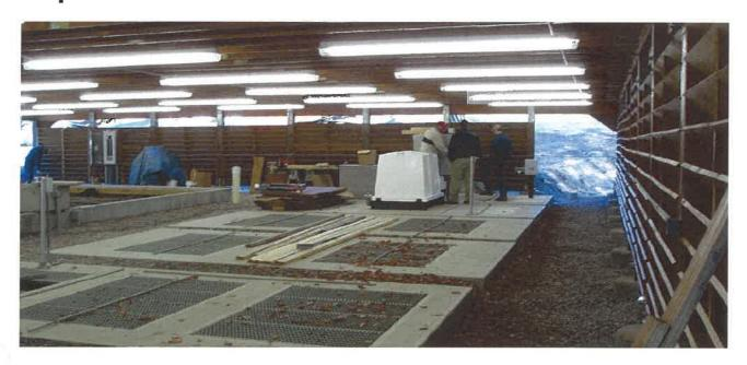
E.L. Robinson Engineering Co. was contracted by the West Virginia Division of Natural Resources, Parks & Recreation to design a new concrete sewage treatment plant which eliminates the potential for rust. The new plant also uses ultraviolet disinfection and provides a sand filter prior to discharge into the Blackwater Canyon.
