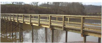
West Virginia Division of Natural Resources received a grant to build a pedestrian bridge approximately 900 feet across the lake from the lodge to the campground. An initial concept plan was developed for the bridge in 2008 which served as the basis of the final design which EL Robinson was retained to develop.
