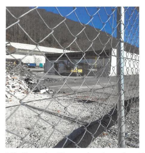
Building 33 was used as a GSD carpenter shop and state mail room. The building footprint was in the way of a medium voltage duct bank require for the building 11 chiller plant expansion. GSD energy di the engineering to remove the carpenter shop half of the building while retaining the State Mail room. The project involved a new electrical service and detailed structural analysis. This project has been successfully completed.
