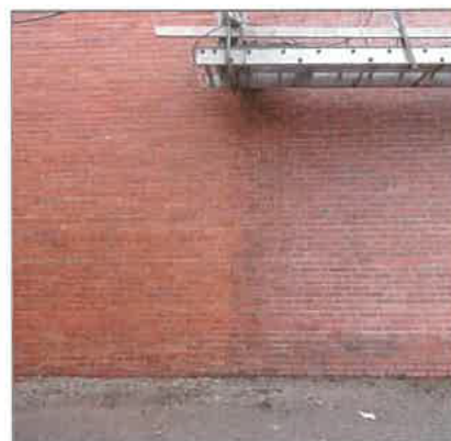
Photo Showcasing Masonry Restoration
