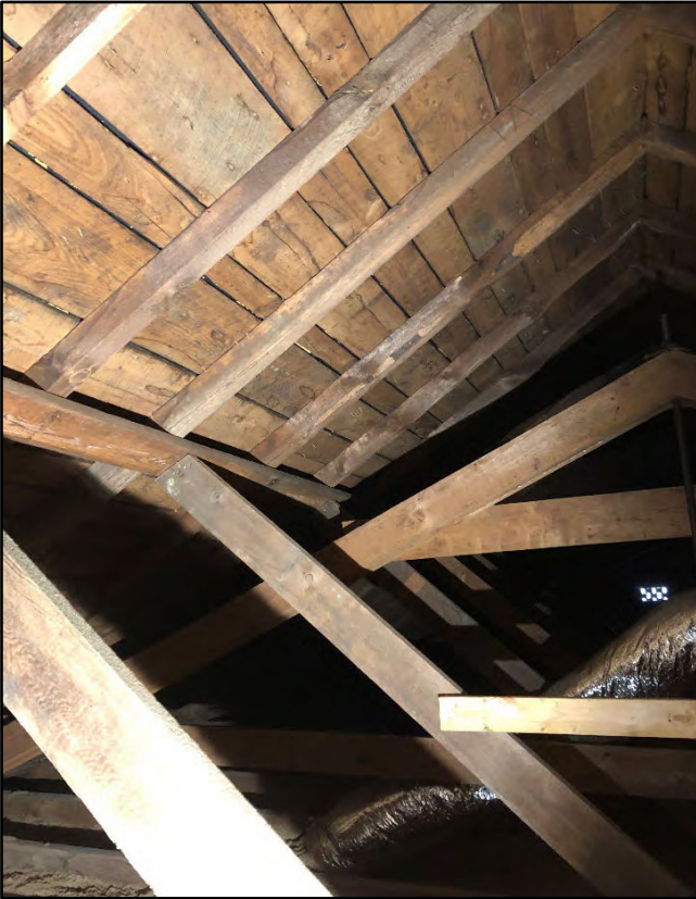
Fig. 012 Underside of existing roof framing
