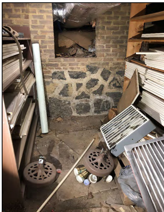
Fig. 002 Note red clay brick formed into mortared together lower basalt stones.
