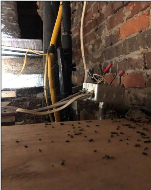
Fig. 014 Attic space over Masonic addition. Notice loose wires.
