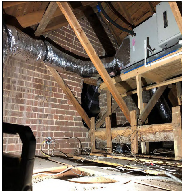
Fig. 015 Open junction box. Notice guano
