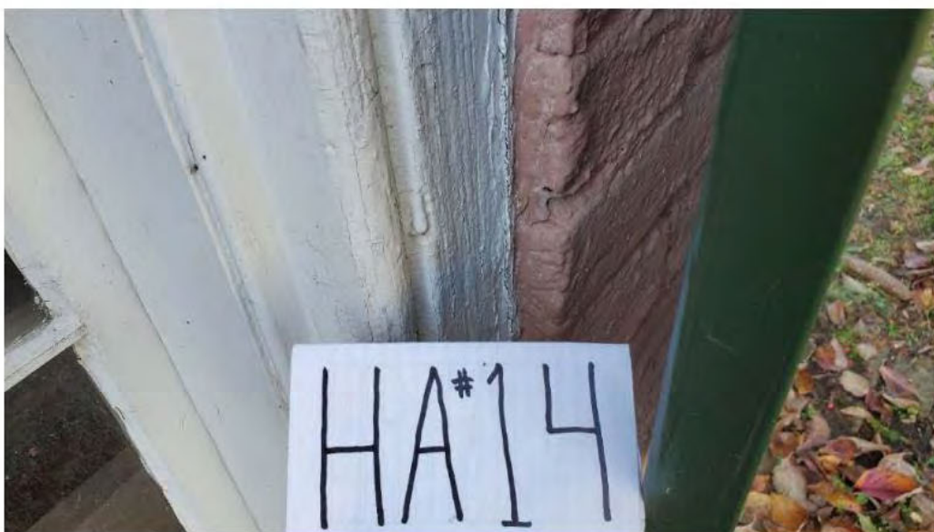
HA #14: Masonry Joint Sealant
