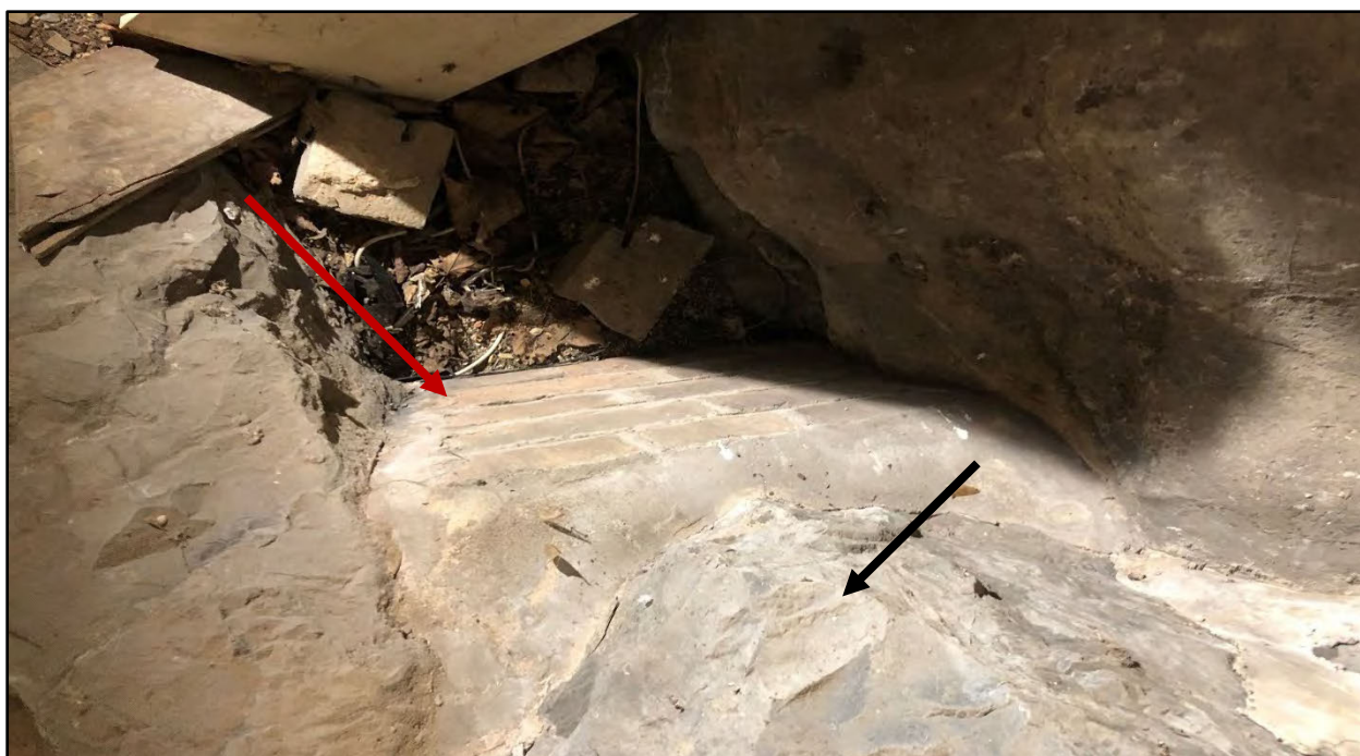
Fig 003 Notice brick support (red) under the footing stone overhang (black).
