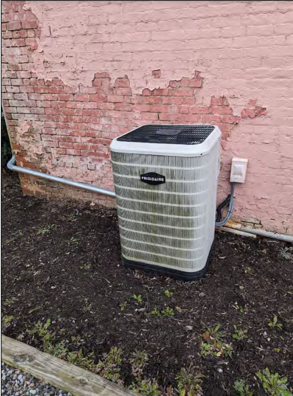
Fig. 044 Outdoor Condensing Unit
