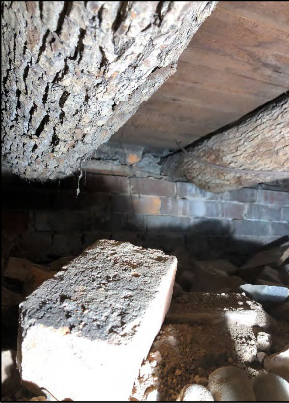
Fig. 008 Footing in original crawl space Note tight space and debris
