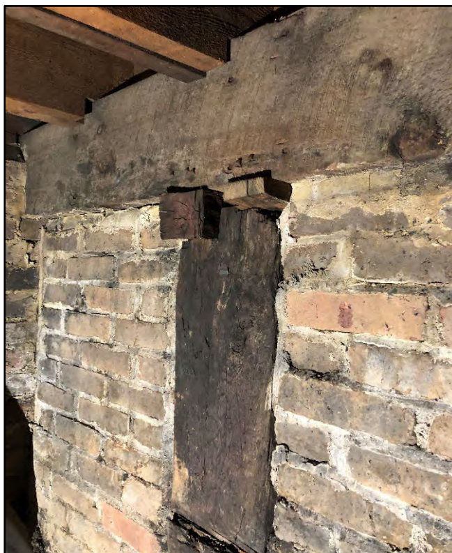
Fig 005 Top, encased column
