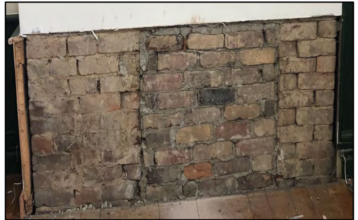
Fig 033 Buried and filled in fireboxes on the second floor
