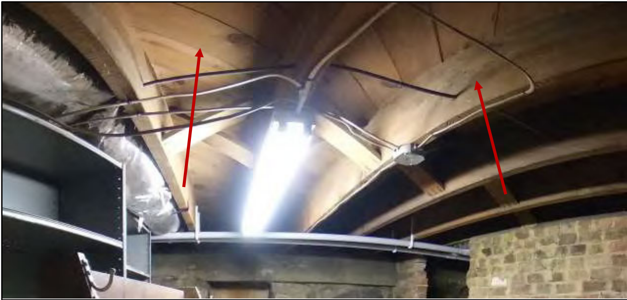
Fig. 011 Framing in the walkable basement. Note modern 2x12 floor joists and diagonal planking.
