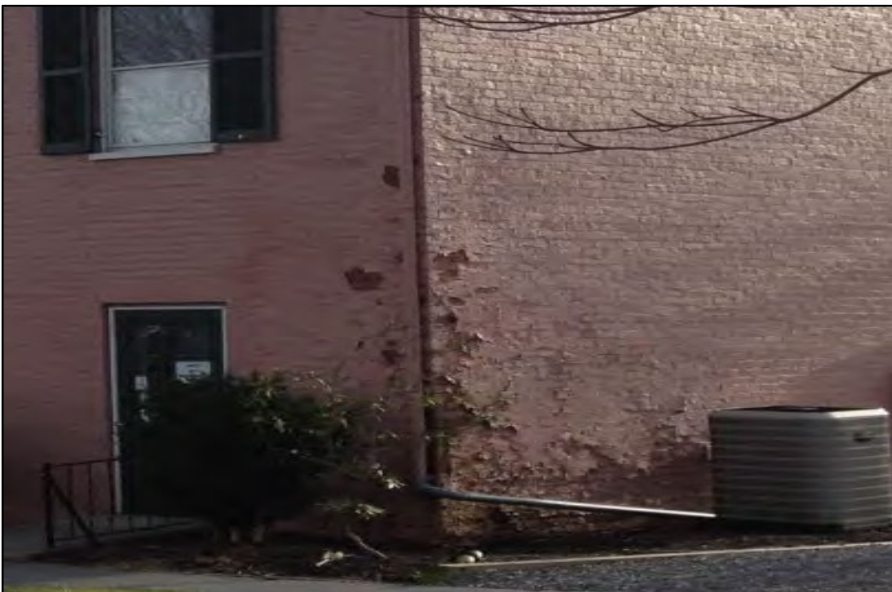
Fig. 016 Northeast exterior corner. Notice deteriorated brick cladding as well as failing paint.
