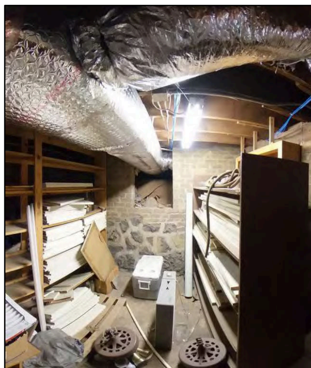
Fig 006 Original north opening to crawl space. Note the finished wall edges
