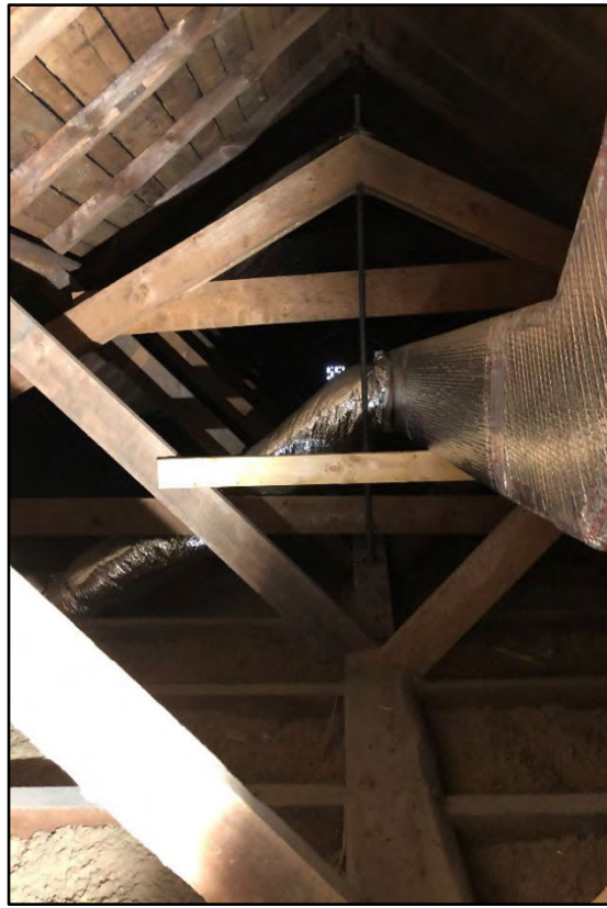
Fig. 013 Modern load-bearing truss attached to the original load-bearing beam
