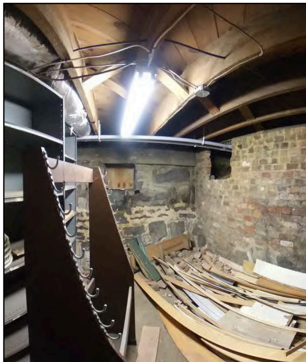
Fig 007 Crawl space access created after original construction. Note broken bricks.
