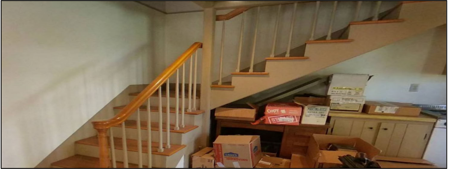
Fig 037 Enslaved Quarters staircase. Note missing Wall handrailing
