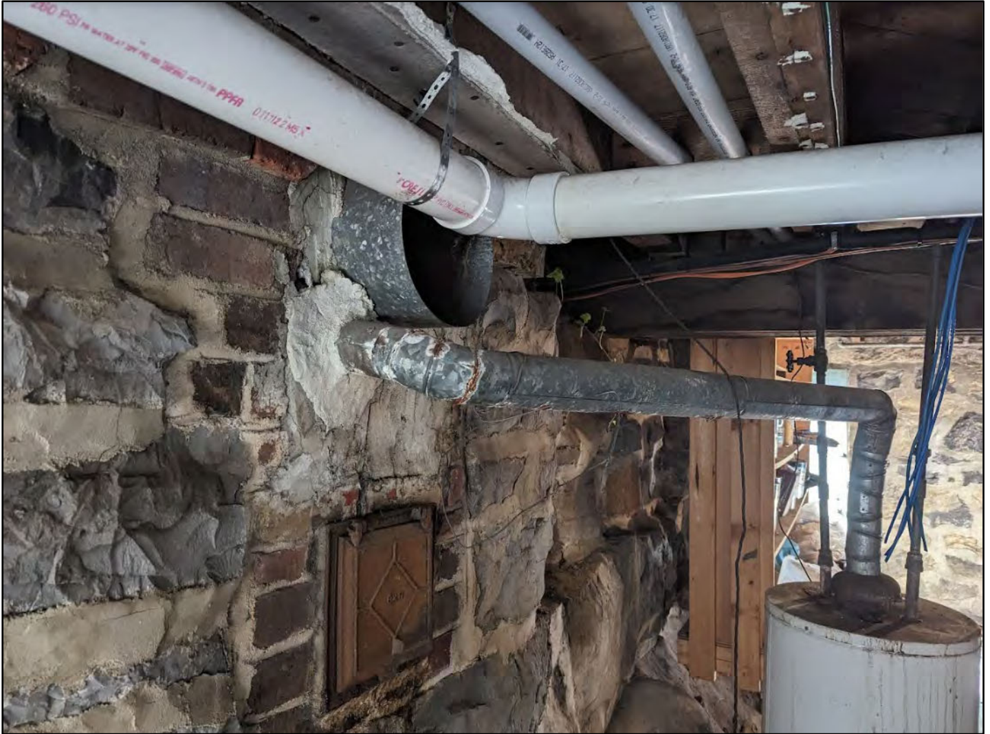
Fig. 048 Water Heater Flue
