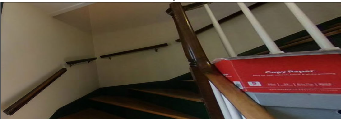
Fig 036 Main building handrail system. Notice noncontinuity
