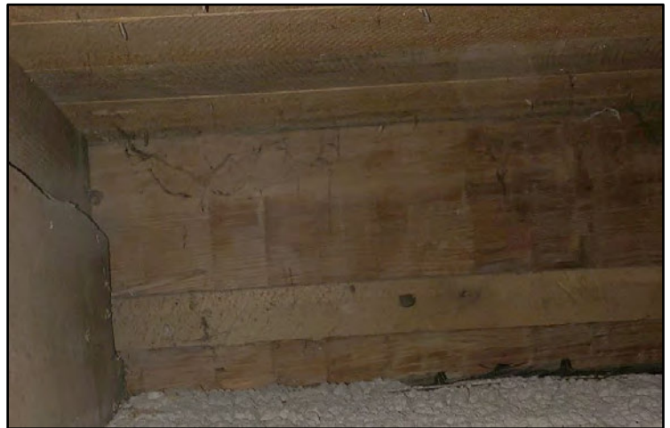
Fig 035 Existing second-floor timber with modern framing attached
