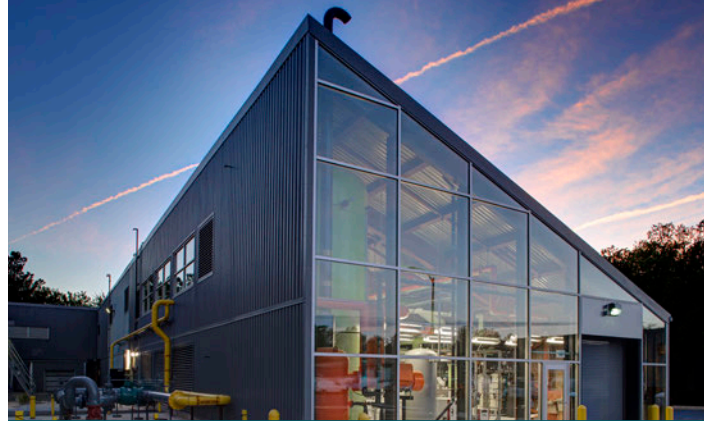
Central Chilled Water Plant Renovation & Expansion George Mason University
