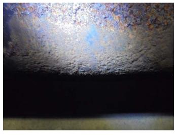
We identified relatively minor surface rust randomly in some areas which, from the above example, can be shown to have had little significant impact against the pipe.
