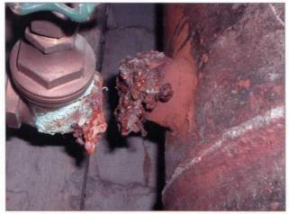
Figure 2. This incidence of corrosion was detected by expanding testing into dead-end areas.
