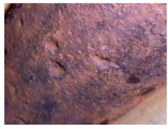
At left we show a closer view of the take-off line at location No. 29 where deep surface pitting is evident having a depth of near 0.045 in. as measured by a surface depth micrometer. Lesser pitting was identified in most other areas of the chill water system in the range typically of near 0.035 in.
