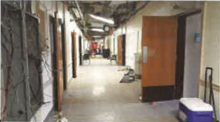
Above: Early Demolition
