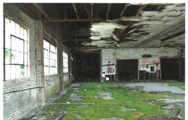
Right: Interior prior to renovation.
