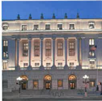
GSA Hipolito Federal Building Location: San Antonio, TX
