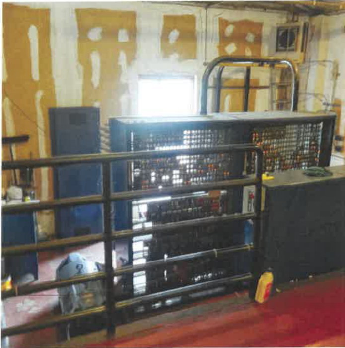
Machine Room Before Modernization
