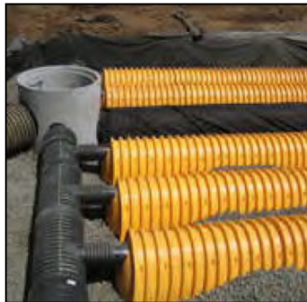
Underground Stormwater Storage
