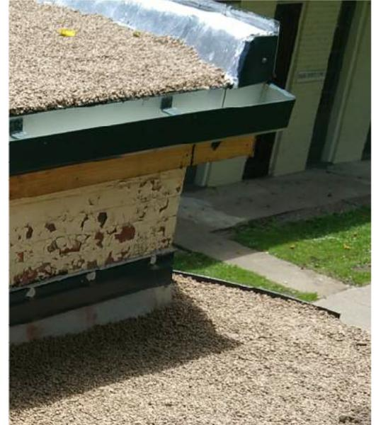
West Virginia Division of Natural Resources contracted Montum Architecture to specify and administer roofing replacement of the Pool Bathhouse at Berkeley Springs State Park. The existing roofing was a combination of EPDM and built-up roofing. Failing wood framing was replaced and ACM abatement was incorporated in the demolition.
