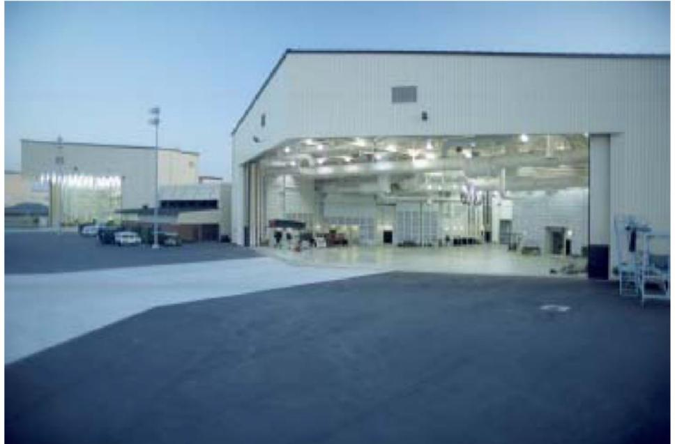
identified activities associated with the B-1B Bomber. The exterior is made of metal panels, reddish brown brick and beige stucco to complement that used on the Joint Starts development across the flightline. Roofs are a dark bronze standing seam metal roof. Exterior windows and doors are dark bronzed anodized aluminum, double glazed.
