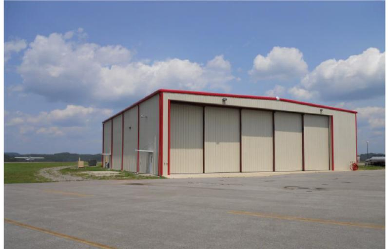
One of the 10,000 SF hangars has an 18-foot door height to accommodate the airport's growing local fixed-based operator; the other hangar has a 28-foot door height for an avionics and interior refurbishing business. A specially-designed reinforced floor slab accommodates a variety of aircraft. Innovative construction details were developed to meet the specific fire safety and building codes while remaining within client's budget.
