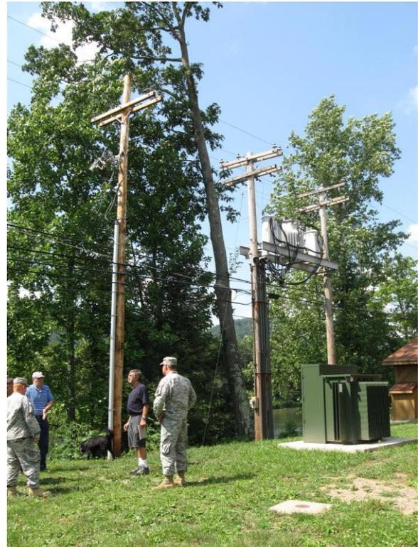
transformers with pad-mounted transformers. The transformers ranged in capacity from 1000 KVA to 50 KVA. Phase 2 included relocating the communications service to new underground duct banks along the same 3000 LF route. The third and fourth phases included the relocation of approximately 2000 LF of overhead power lines and overhead communications lines to new duct banks, respectively. Vacuum interrupters were added to improve selective coordination between various circuits.
