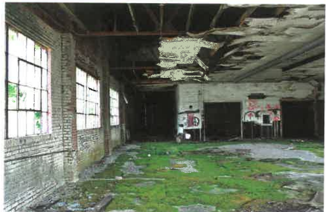
Right: Interior prior to renovation.
