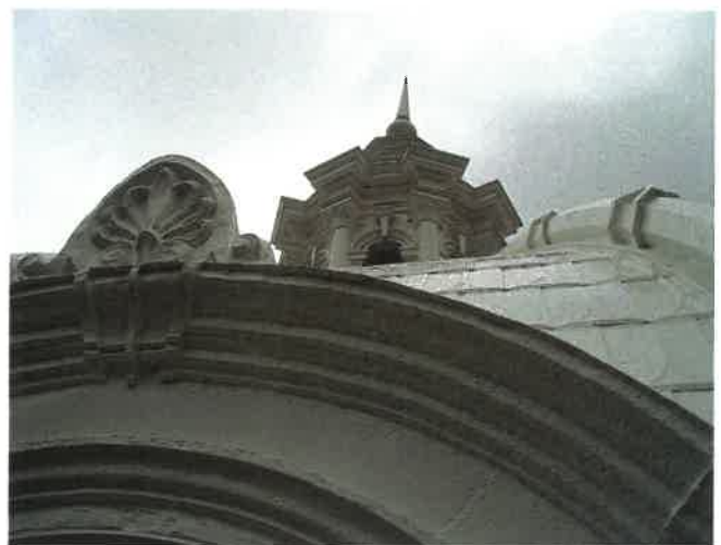
Dome Restoration Detail
