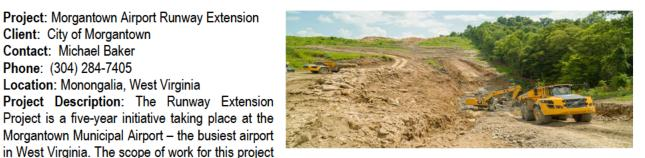
is to extend the existing runway by 1,001 feet, creating a safer takeoff and landing space for outgoing and incoming flights. Over 100,000 CY of rock excavation was part of the scope of the PH-1 project.
