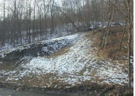
strata depths and water levels, using piezometers. Slope stability analyses were performed to determine the corrective actions required to stabilize the area. Surface and subsurface drainage structures, a too key, and stream bank protection were designed to correct the instability
