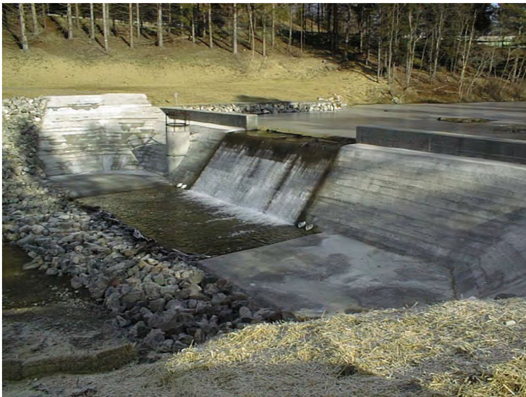
THOMAS DAM MODIFICATION, THOMAS, WV
