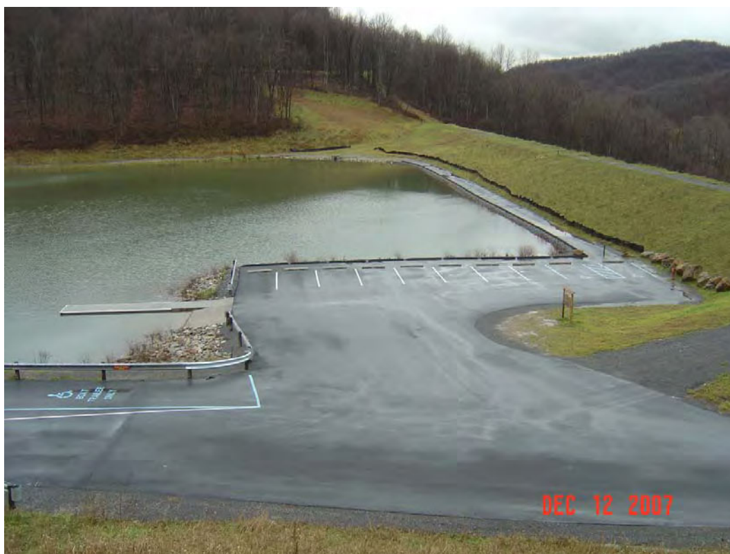
BAILEY DAM MODIFICATION, MONONGALIA CO., WV
