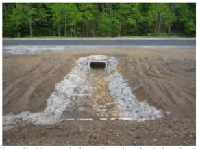
POTESTA provided a survey crew and engineer that selected and staked proposed drainage channels and culverts in the field. Utilizing the survey information, POTESTA prepared plan view drawings, channel and culvert profiles, and details depicting the proposed abatement measures to control surface water and minimize erosion.
