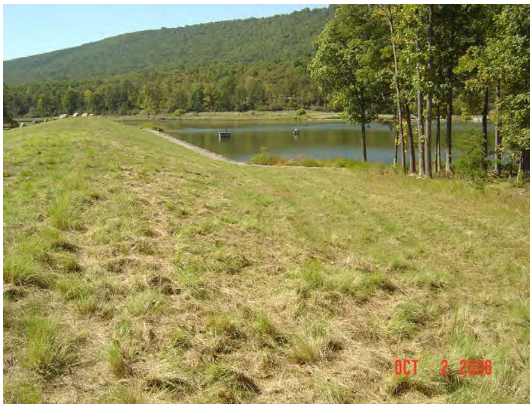
WARDEN LAKE DAM MODIFICATION, HARDY CO., WV
