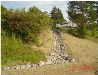
**Erosion Repair – Rip Rap Armored Ditch**
