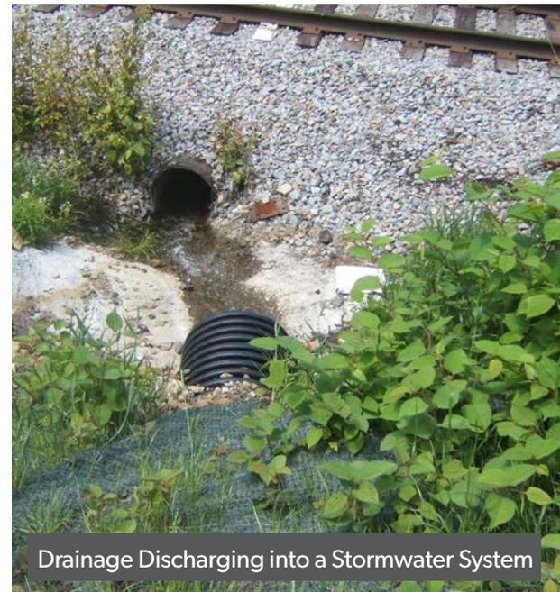
Drainage Discharging into a Stormwater System
