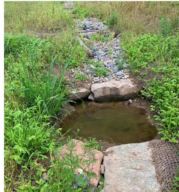
GAI developed and prepared a stream restoration plan with necessary plan sheets to fulfill the Client's obligations of restoring and monitoring approximately 450 linear feet of ephemeral and intermittent stream. Stream restoration involved reestablishment of channel in a previously filled valley. All streams will be restored to stable pattern, dimension, and profile, providing increased bedform diversity, sediment, transport, and biological lift.
