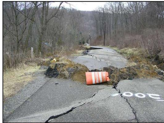
Site design will begin on the collection and diversion of ground water, slope stability and road replacement once the final site investigation has been completed.
