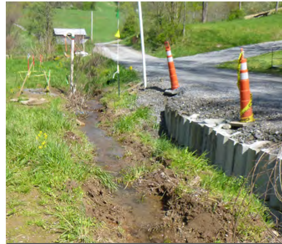
Impacted Stream Before Construction
