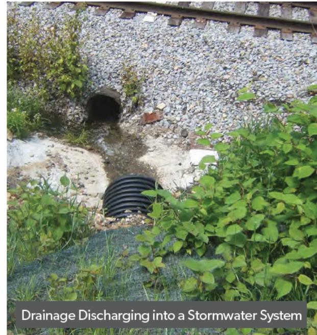
Drainage Discharging into a Stormwater System
