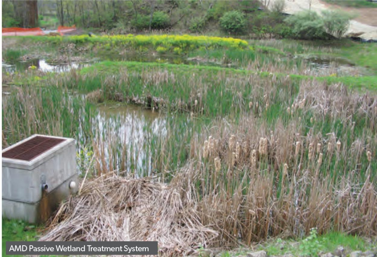
GAI designed, permitted, and prepared construction plans for the collection and passive treatment of AMD surface seepage from nine hillside seeps. The seepage was emanating from the abandoned mines located on our Client's property near Shelocta, Pennsylvania. The purpose was to clean up AMD seepage that was mixing with stormwater runoff and discharging at existing station NPDES Stormwater Points.
