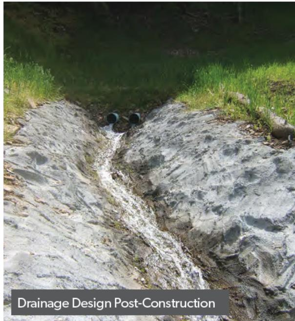
Drainage Design Post-Construction
