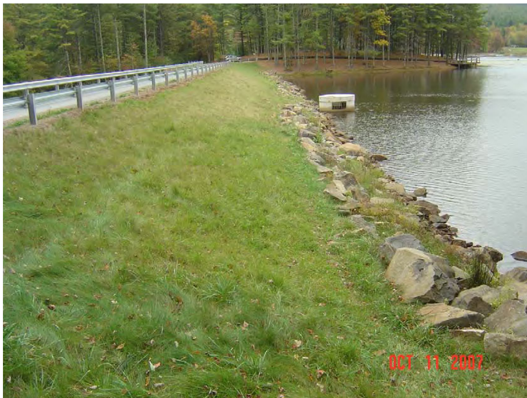
MONCOVE DAM MODIFICATION, MONROE CO., WV
