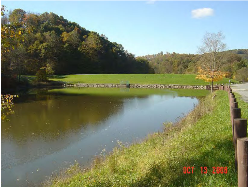
JIMMY LEWIS DAM MODIFICATION, MERCER CO., WV
