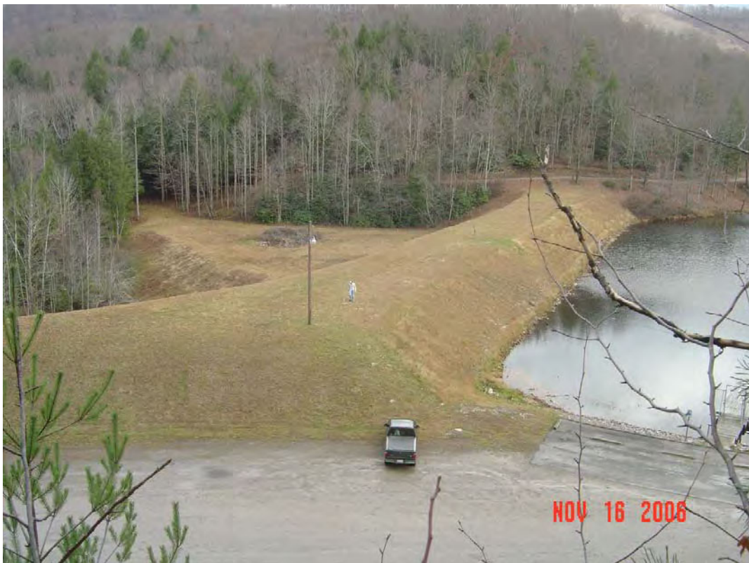
PLUM ORCHARD DAM MODIFICATION, FAYETTE CO., WV
