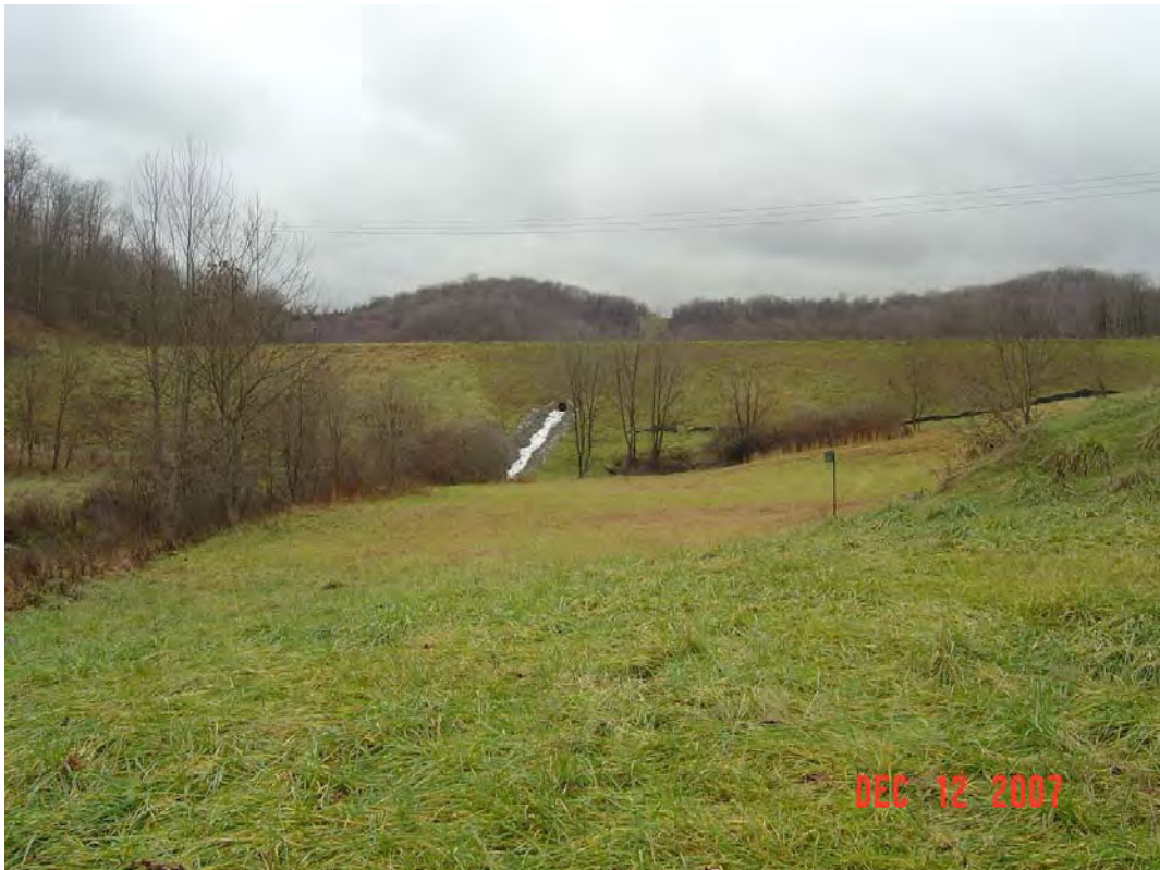
LEMLEY DAM MODIFICATION, MONONGALIA CO., WV
