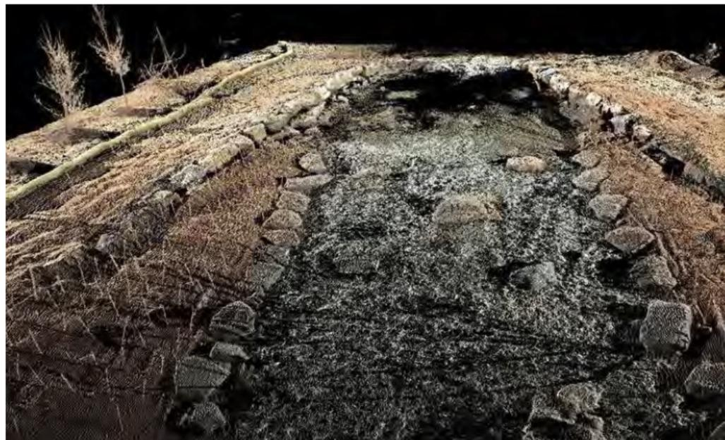
*3D As-Built Scan of a Cross Vane*
