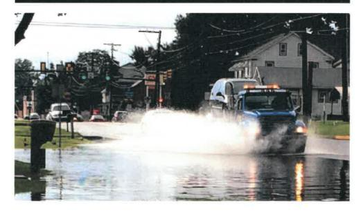
capacity. The combination of the large contributory area, flat topography and undersized conveyance system led to flooding of the road in even short, but intense, storm events. The extent of road inundation results in hazardous driving conditions that mandate intervention.
