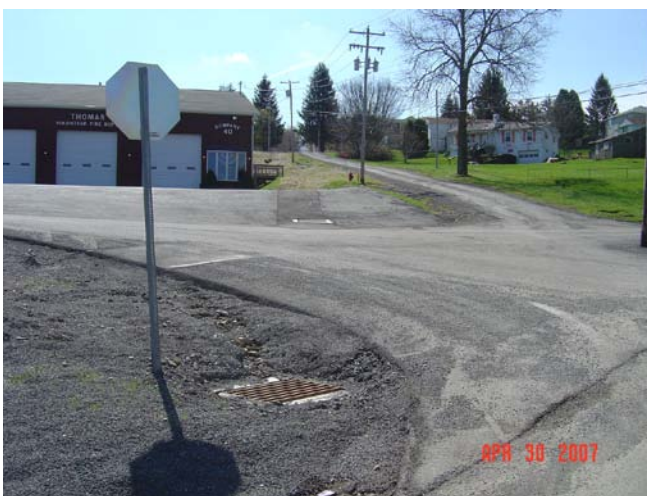
New Storm Drains and Catch Basins
