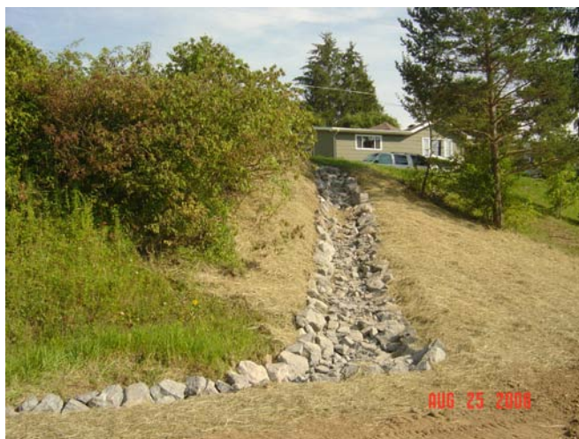
Erosion Repair – Rip Rap Armored Ditch
