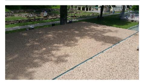
West Virginia Division of Natural Resources contracted Montum Architecture to specify and administer roofing replacement of the Pool Bathhouse at Berkeley Springs State Park. The existing roofing was a combination of EPDM and built-up roofing. Failing wood framing was replaced and ACM abatement was incorporated in the demolition.
